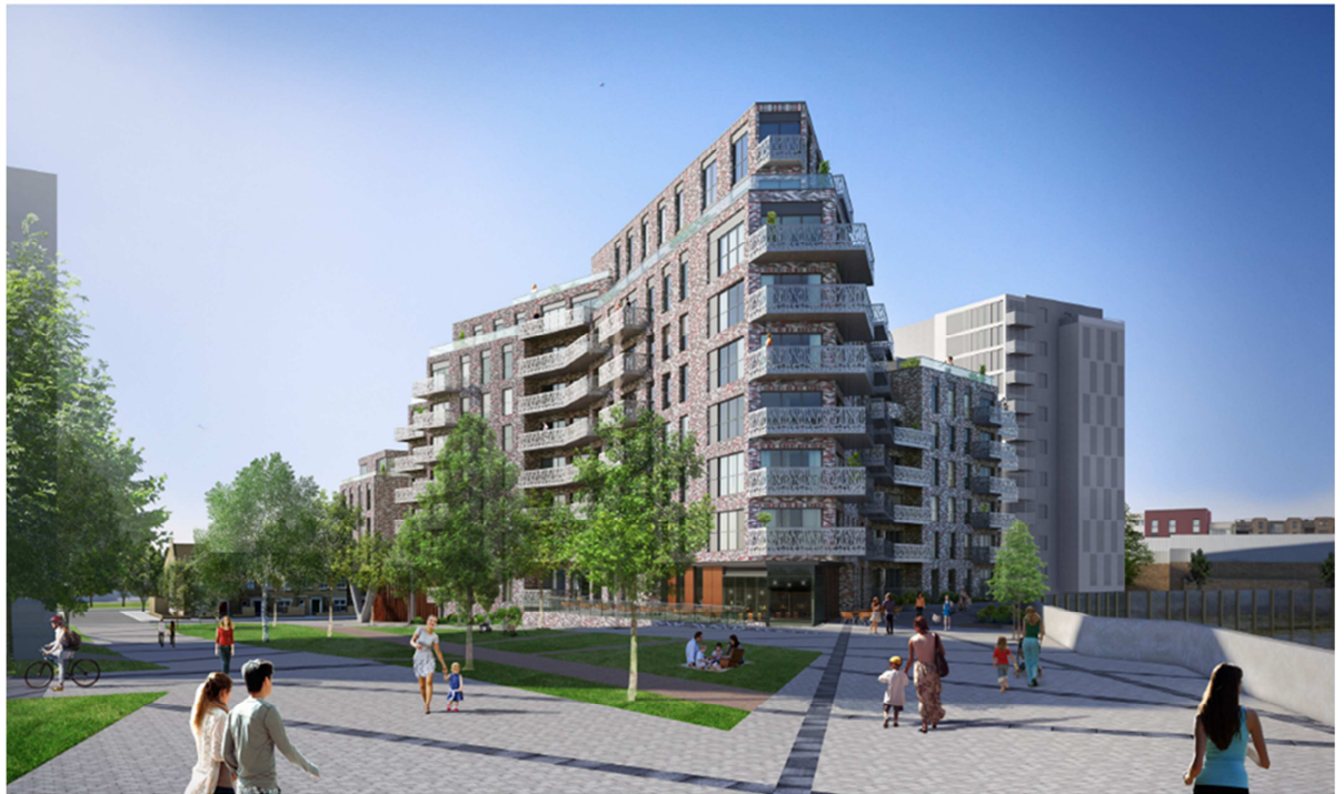
Figure 3 View of the proposed development from neighbouring gas works site (by the riverside) showing the riverside ground floor flexible floor space located at the apex of the 9 storey Block A. The under construction Devon's Wharf scheme (which is 11 storeys) is also shown abutting the proposed development towards the right edge of this image)
